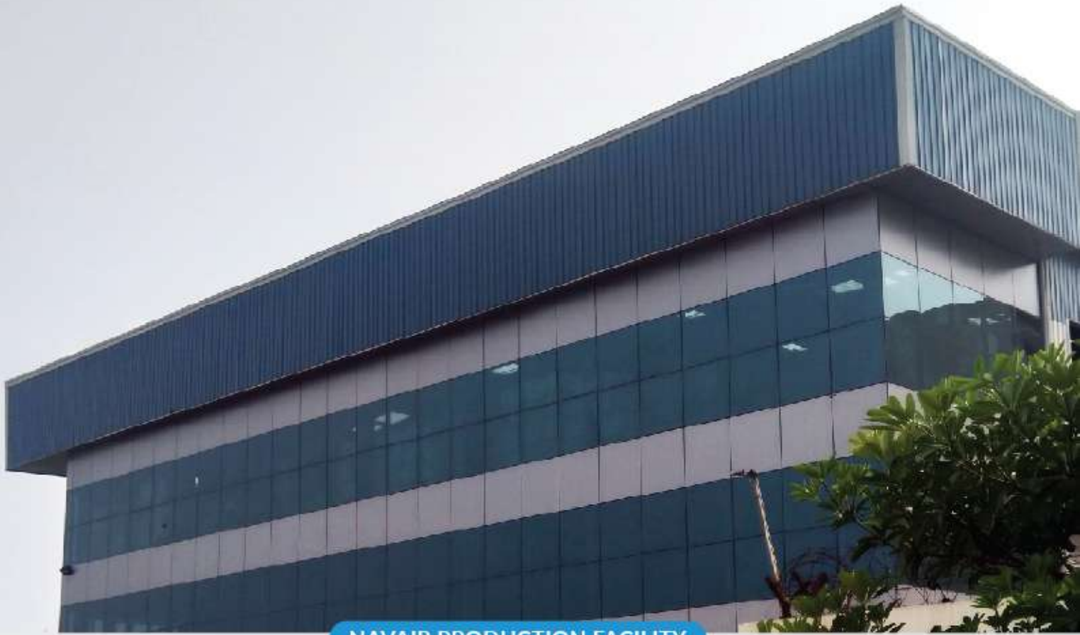
NAVAIR PRODUCTION FACILITY
